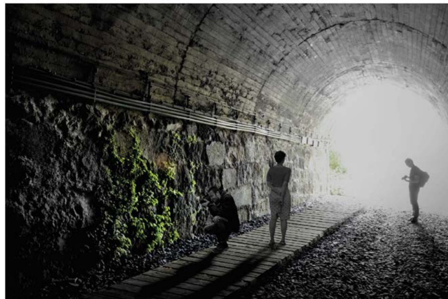
THE ENTRANCE TO THE TUNNEL
