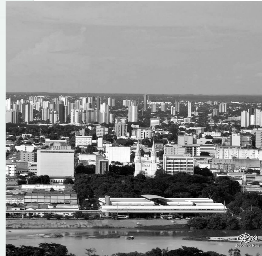
Physical barriers (train station and a mall) separate the river landscape from the square.
