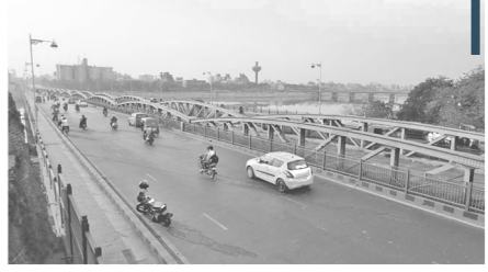
Ellis Bridge - current state
