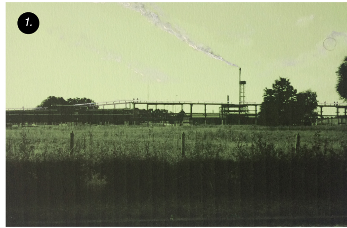
new public route on existing pipe columns
