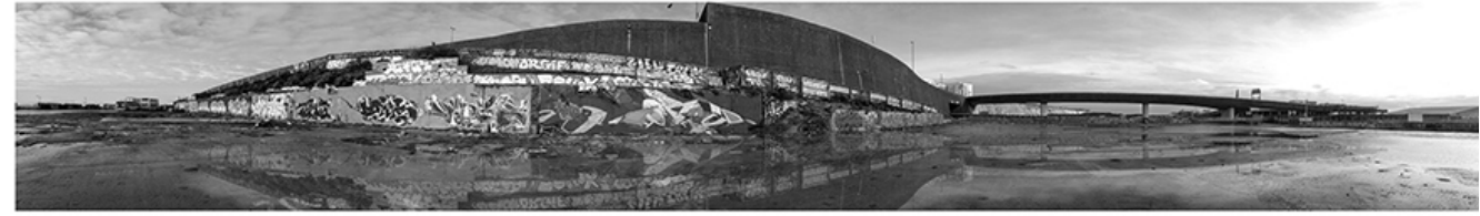
Polluted Surface water accumulation
