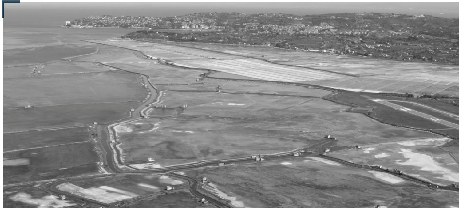
Current state of the salt pans showing the deteriorated area of the medieval salt production.
