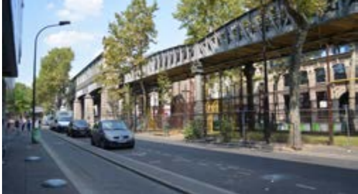
Barriers under the Viaducts space
