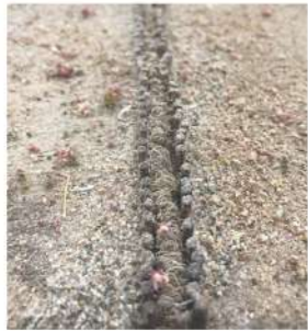
Detail model: double raw of wooden poles filled with branches lets the water pass and traps the sediments. Opposite to a normal groyne, its permeability allows for uniformity of sedimentation.
