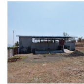
I4: Adhoc structures built, poor land planning.
