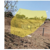
I1: Irregular grading of site and poor soil. Current grading can cause top soil erosion.
