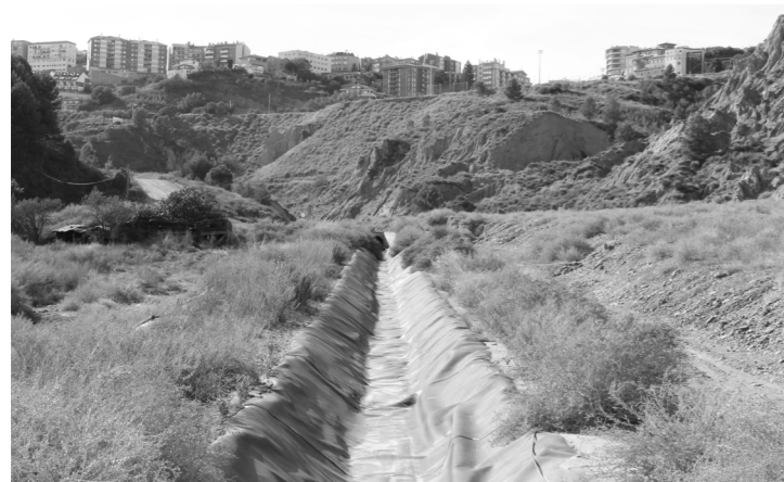
Drainage ditch in the Saline Valley.
