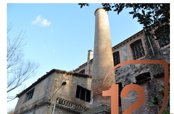
View of the chimney
