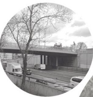
Actual view of the bridge
