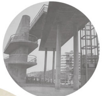
Actual view of the bridge
