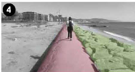
4 Presence of breakwater and sewage collector on the coastline
